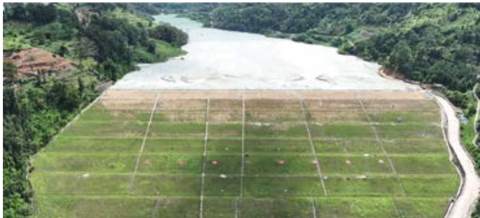
Tailings storage facility of Malipo Zijin Tungsten
